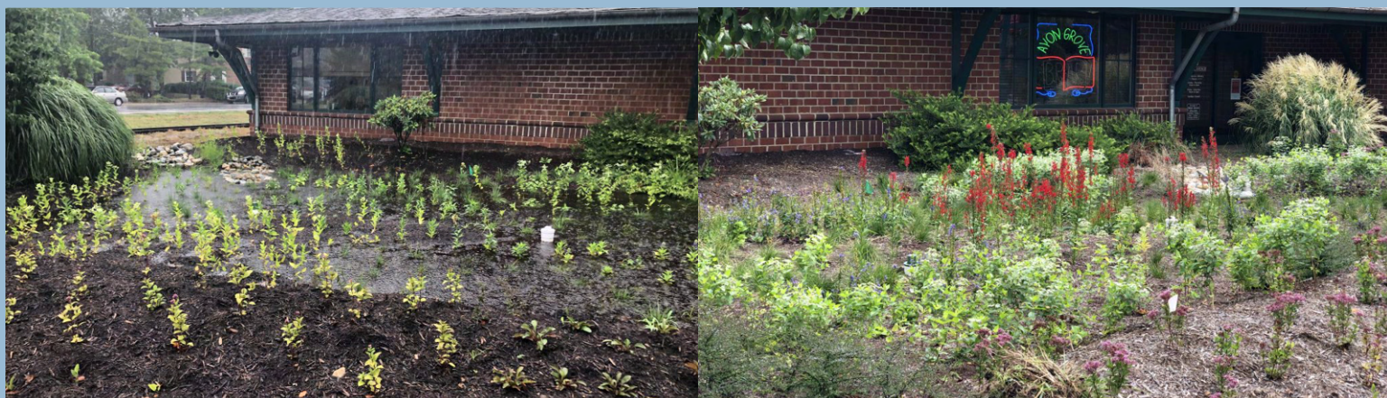
On the left is a recently installed rain garden full of stormwater during a two-inch rain storm in July 2020. On the right is the rain garden in bloom three months after installation.
