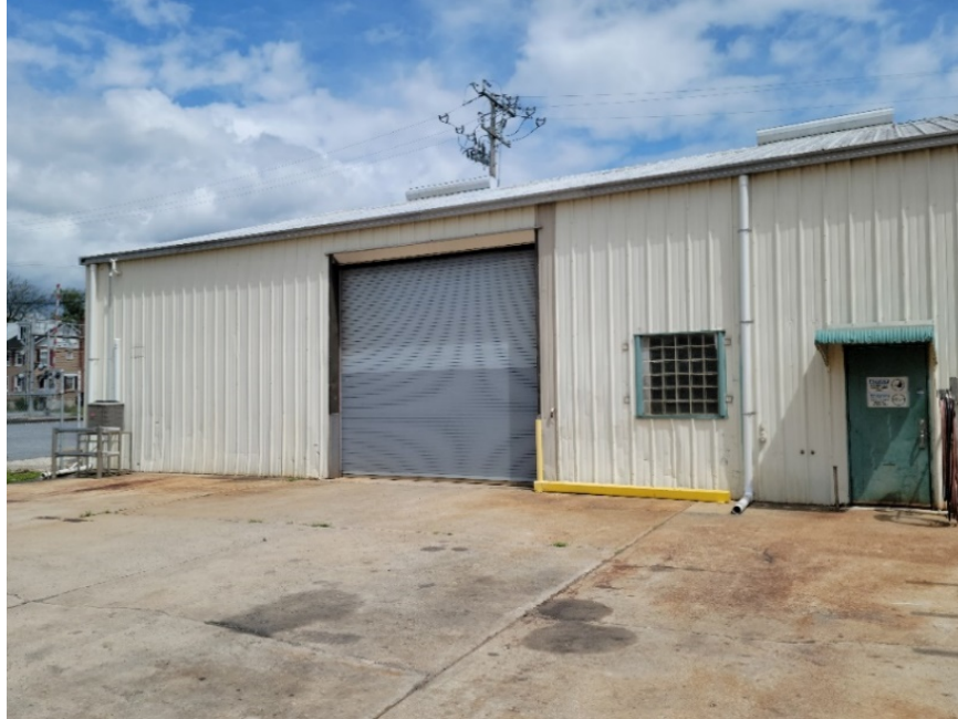
The exterior of the proposed Kennett Fire and EMS Regional repair and maintenance shop.
