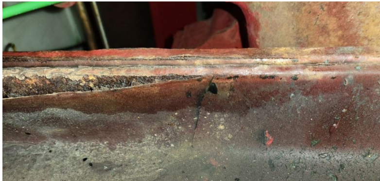
The underside shows moderate to severe corrosion and would need to be repaired if the vehicle is not removed from the fleet.
