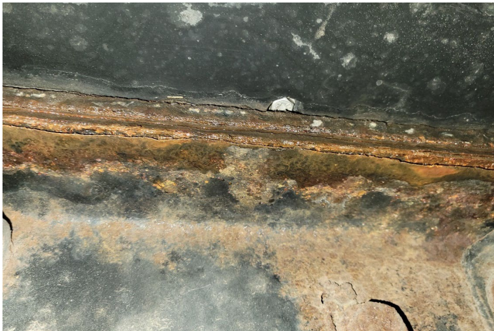
Remediate rust and corrosion on Tanker 25-1
