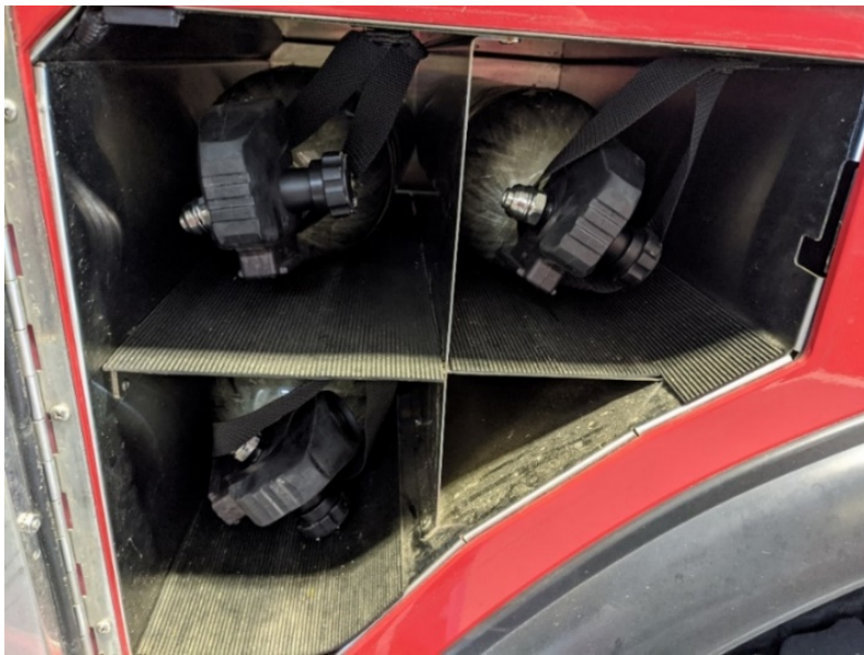
Wheel well compartment showing signs of dirt intrusion. Compartment needs to be cleaned and gasket inspected and replaced.
