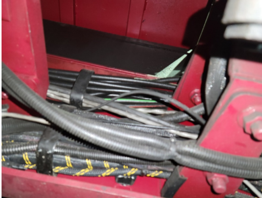
Painting underside components helps protect them from corrosion
