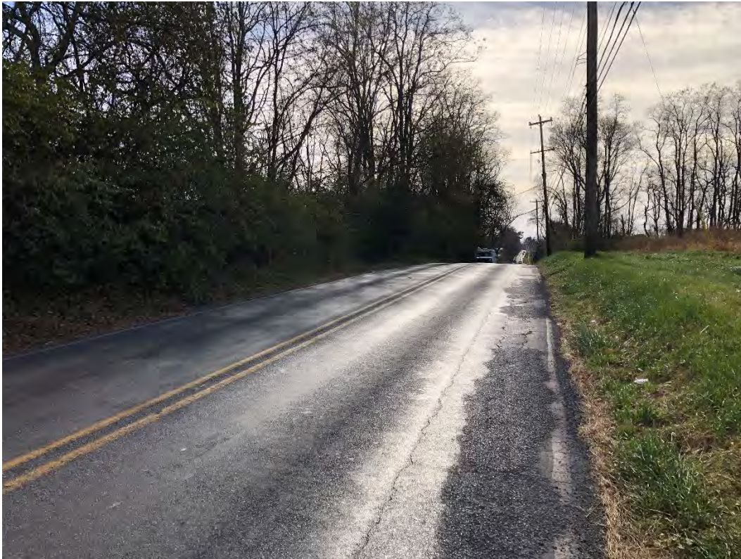
Field View 9: Kaolin Road View, exiting the intersection.
