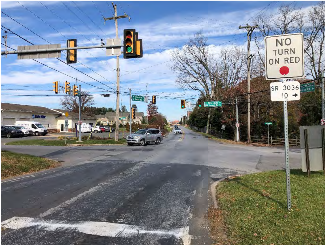
Field View 2: Kaolin Road View, entering the intersection from the northbound approach.
